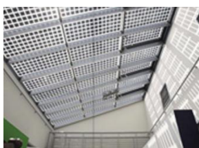
4-rasm. Shisha sirtiga surtiladigan lyuminessent konsentratorlari mavjud quyosh panellari.
